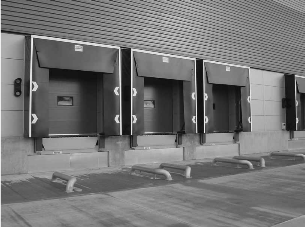
Figure 20.3 Raised dock loading bays
