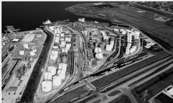
FIGURE 3.4 Odfjell Terminals, Houston (Texas, USA). (Courtesy of Odfjell Tankers.)
