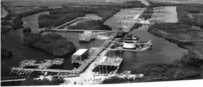
FIGURE 11.5 Louisiana Offshore Oil Port (LOOP). (Courtesy of LOOP LLC.)
