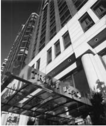
Trump Place on Manhattan's Upper West Side, 180 Riverside Drive.
