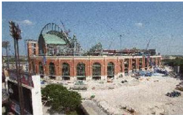
Figure 19.4 Extensive Damage to Stadium After Collapse
