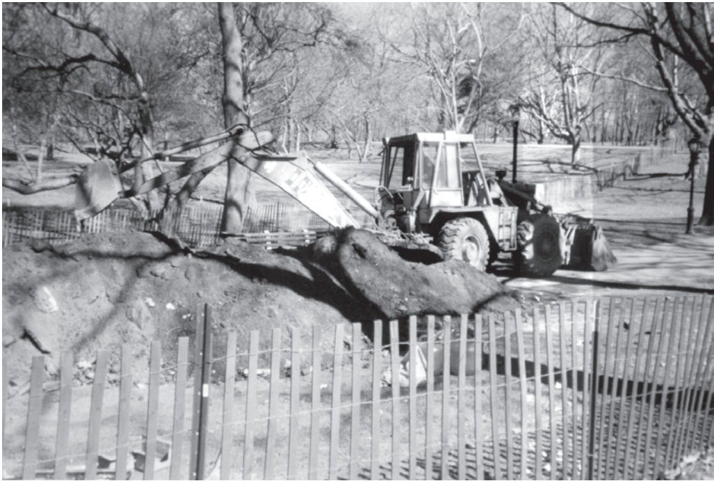
Figure 2.1C A Bulldozer as the Ultimate Tool
