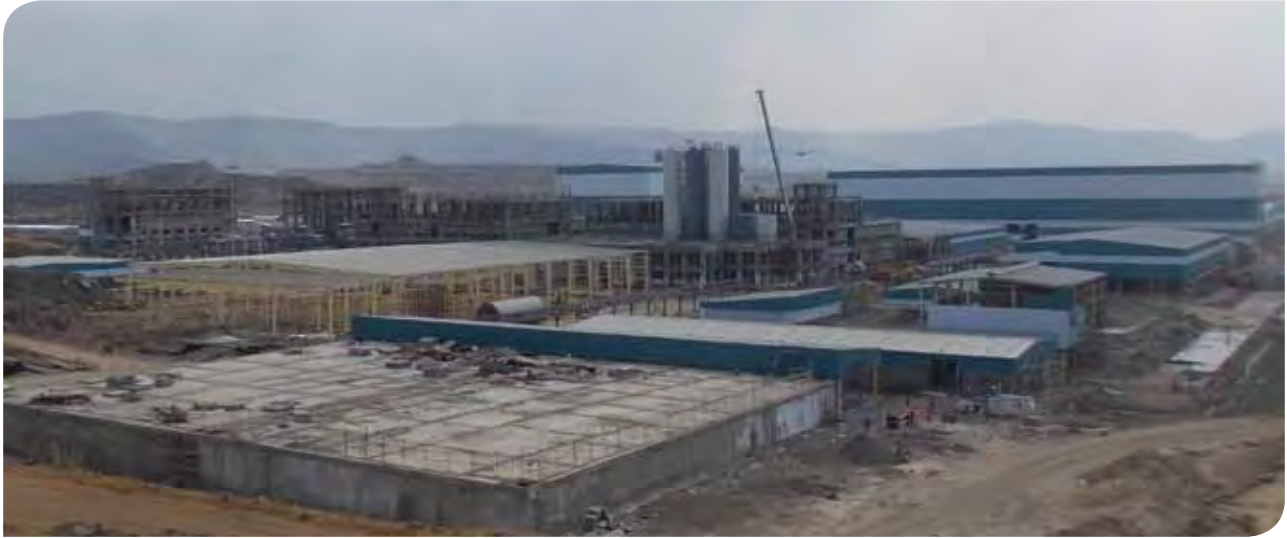
Khandala plant under construction
