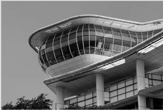
FIGURE 8.1 NLB's National Library Building Is a Prominent Landmark Located in the Heart of the Cultural, Entertainment, and Civic District of Singapore
