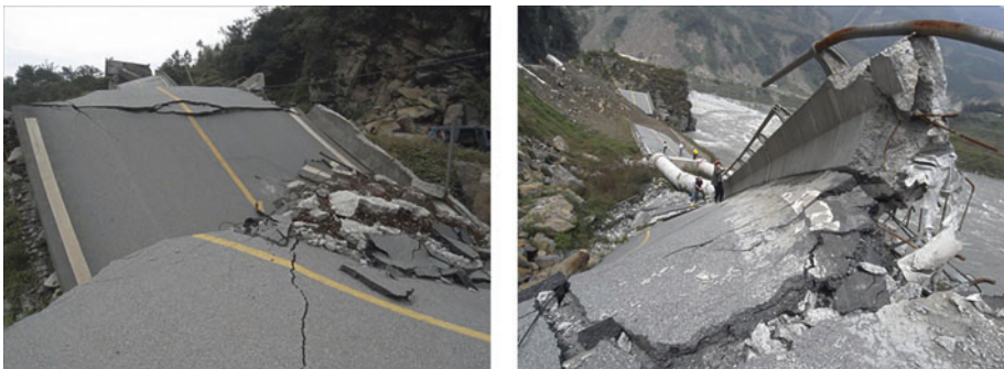
Fig. 18.1 Examples of severe route damage, Nepal 2015 (Source: Quanjing, 2016)
