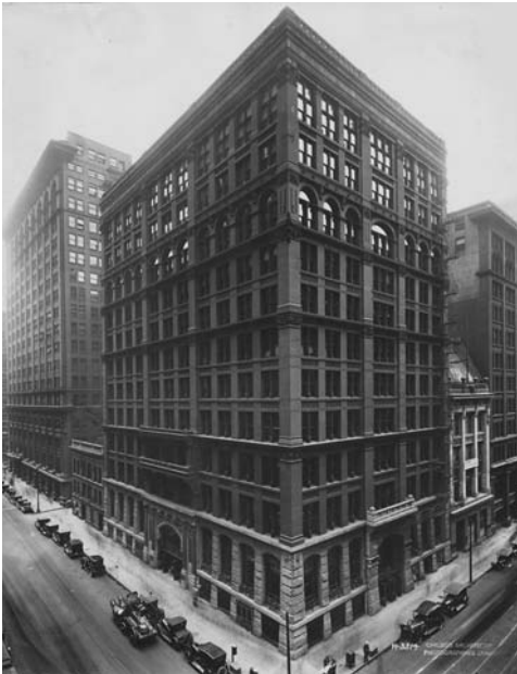
The world's first skyscraper—the Home Insurance Building in Chicago. (Chicago History Museum/Getty Images)
