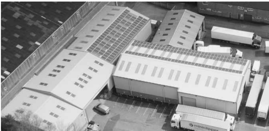
FIGURE 16.3 Solar panels on warehouse roof (courtesy of Miniclipper)
