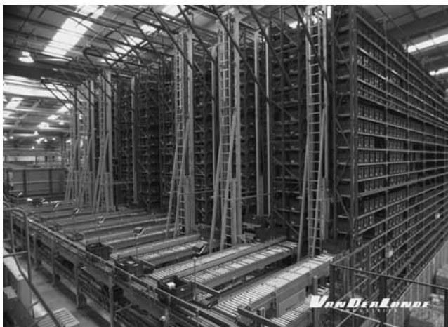
FIGURE 5.3 Mini-load system (courtesy of Vanderlande)
