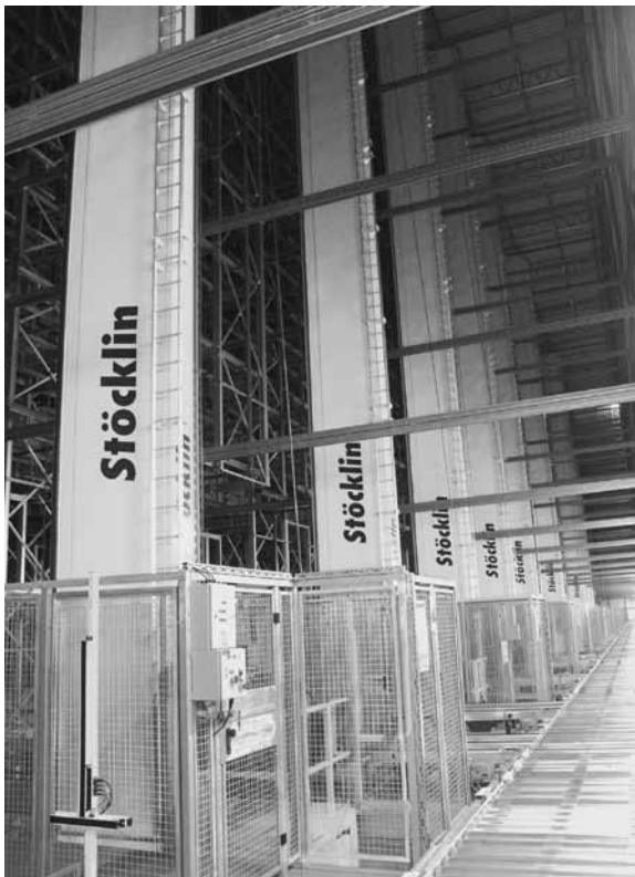
FIGURE 10.23 Crane system for AS/RS (courtesy of Stöcklin Logistik)
