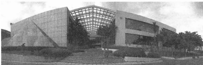
The Infosys Leadership Institute headquarters building in Mysore
