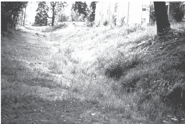
This is a natural well vegetated biofiltration facility. It is not regularly mowed but is performing its water quality function.
