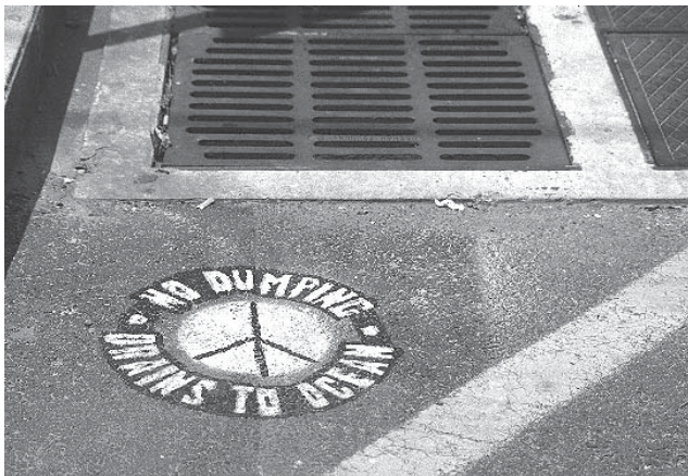
Stenciled pollution message adjacent to a filtration facility.
