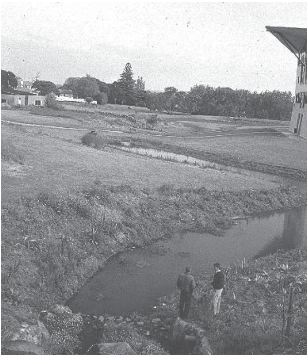
Example of a forebay prior to flow entering the wet pond, which is located in the rear of the picture.
