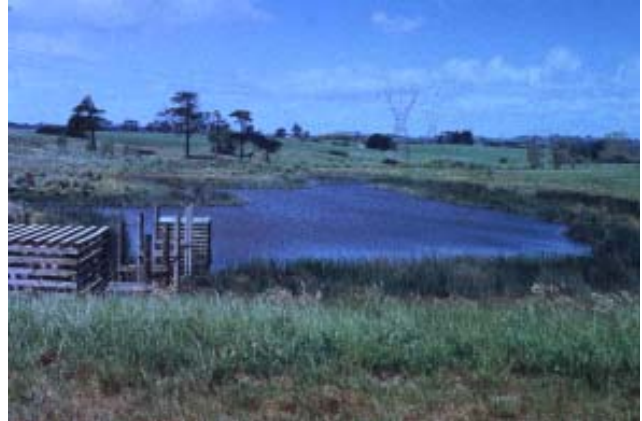
Constructed wetland serving a residential community showing good site stabilization.
