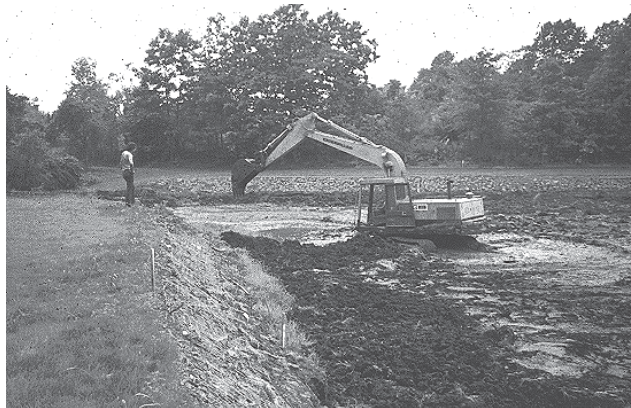
Sediment cleanout of a stormwater management pond.
