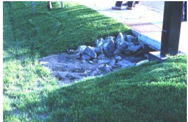
Swale inlet energy dissipator and flow spreader.
