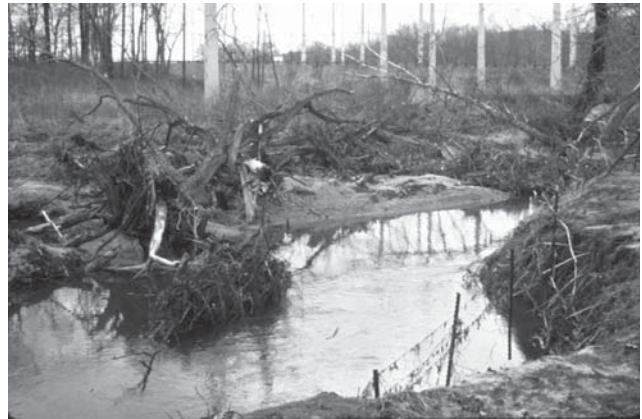
Increased channel erosion in an urban environment.
