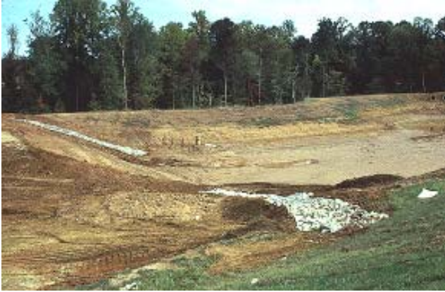
Example of an infiltration basin being constructed.
