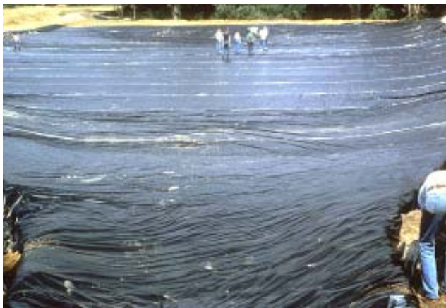
Geotextile liner for a constructed wetland.
