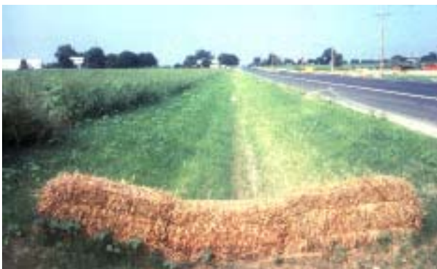
The same biofiltration swale with permanent vegetative stabilization three weeks later.
