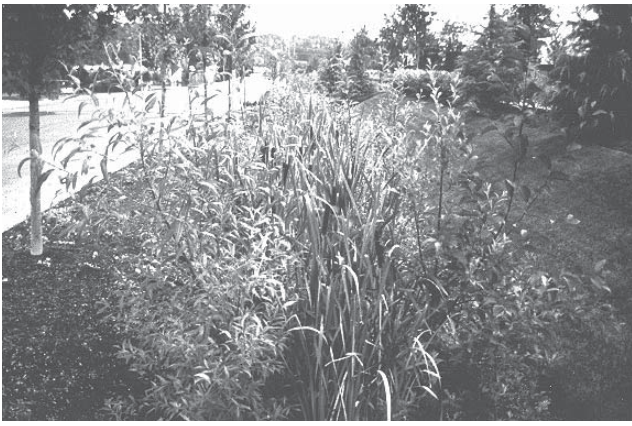
Biofiltration swale with little slope, poor drainage, and baseflow. The swale is well vegetated with wetland plants.
