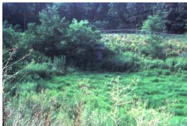
Woody vegetation growing on a pond embankment because of a lack of mowing.
