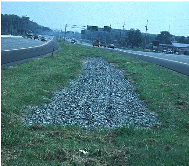
Example of an infiltration trench treating highway runoff.
