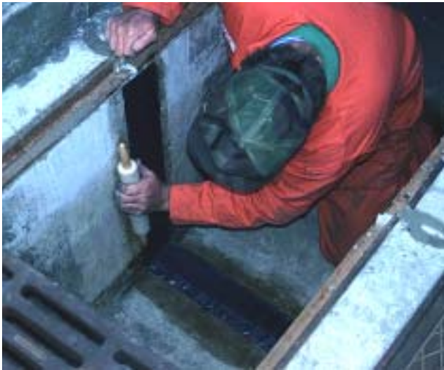
Sealing of joints on a prefabricated Delaware sand filter.
