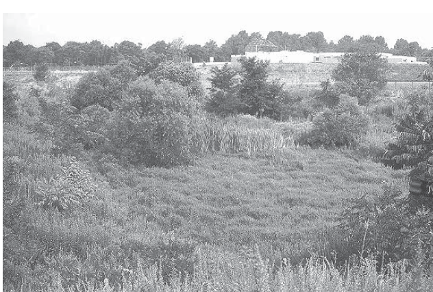
Example of trees all around the detention facility perimeter. It is obvious that maintenance has not been done in years.
