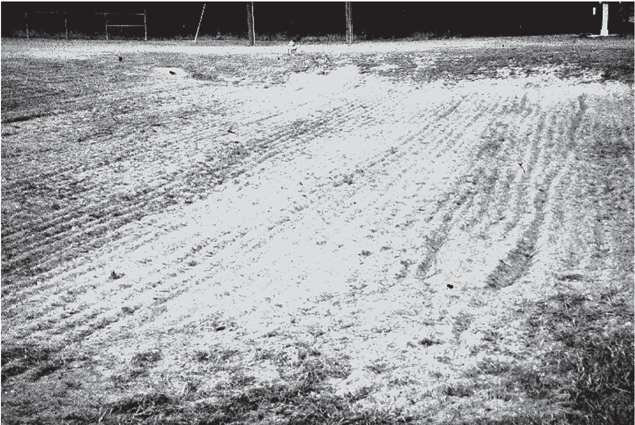
A retention basin which has been recently tilled to help restore its infiltration capabilities.
