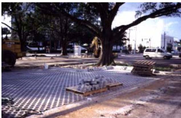
Turf block parking lot under construction.
