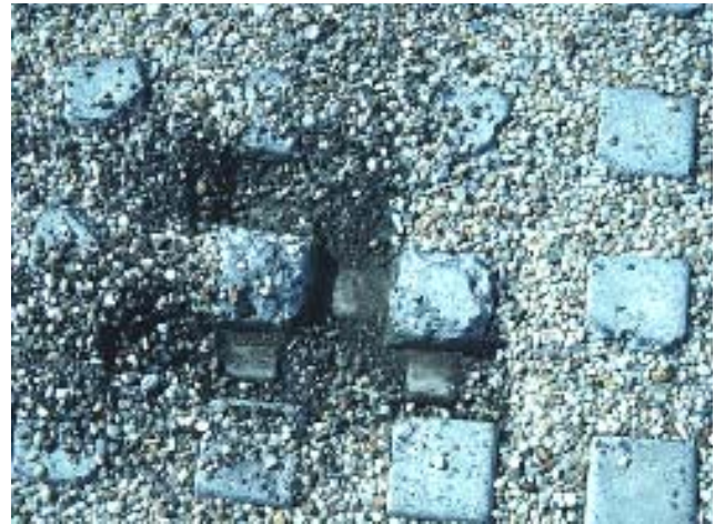
Close-up view of lattice block paving with pea gravel filler in the porous areas.
