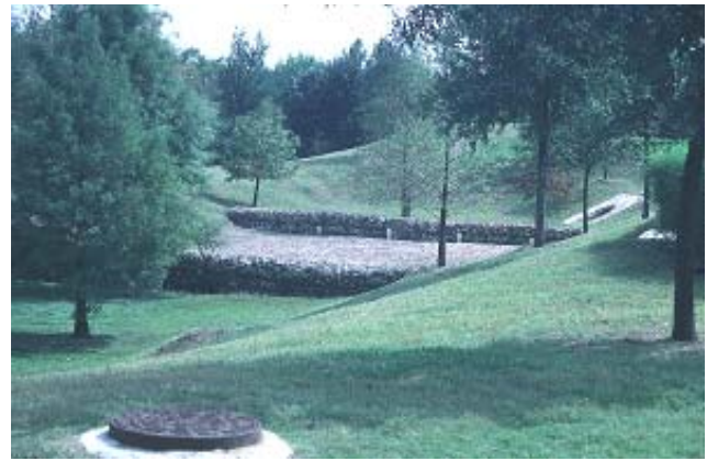
Austin sand filter system sediment forebays on either side with sand filter in the center.
