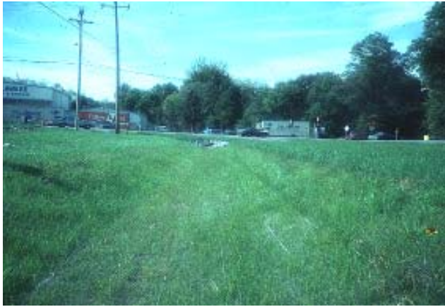
Vegetative swale functioning as a biofiltration facility.
