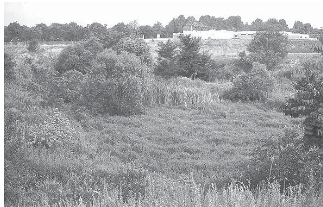
Trees in this stormwater detention basin are an indication that aesthetic maintenance has not been accomplished.
