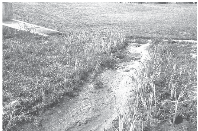
Potential mosquito habitat resulting from inadequate drainage.
