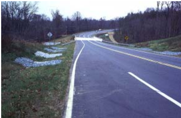
Infiltration swale adjacent to a highway.
