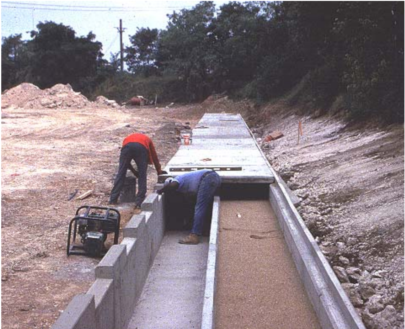
Delaware sand filter being installed in Alexandria, Virginia.
