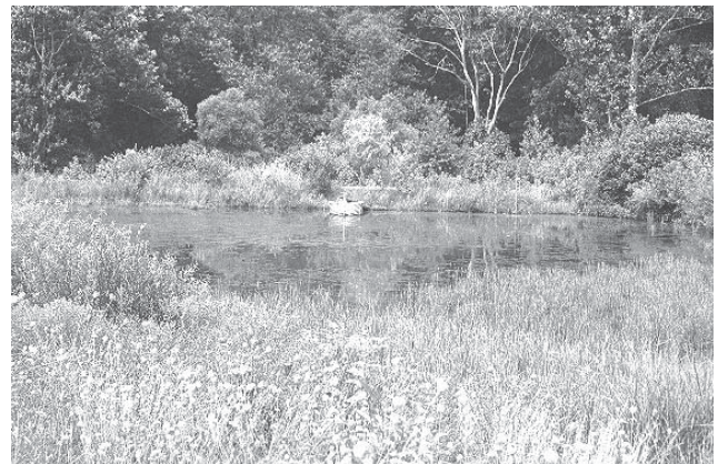
A constructed wetland without sediment forebays filling in. This facility is about 10 years old and will need to be dredged of sediments within the next 10 years. Constructed wetlands are very susceptible to filling in if inflow sediments are significant.
