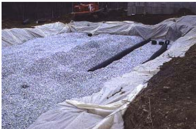
Placement of the reservoir base at a porous pavement site.
