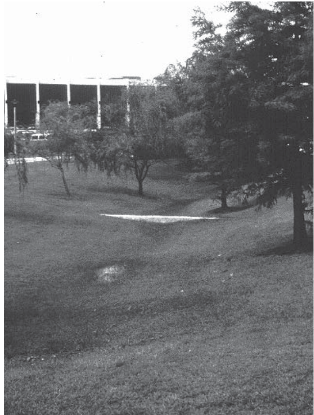
Swale with a swale block.
