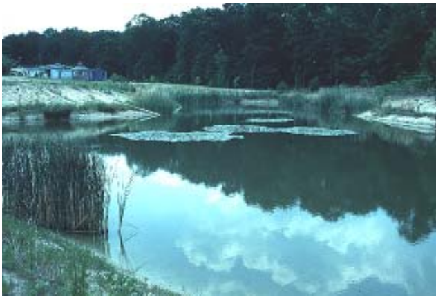
Combination detention facility and infiltration basin where exfiltration from basin occurs through the side walls.
