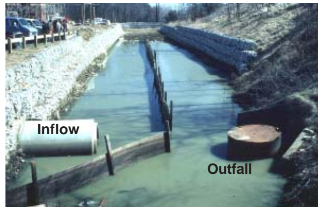
An example of a pond inflow point being close to the outfall.
