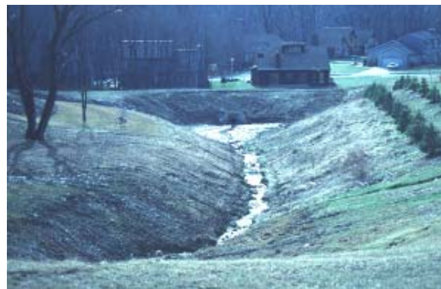
Steep side slopes at a dry pond. Note playground equipment at left top of slope.
