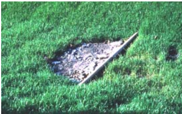
Check dam with energy dissipator.
