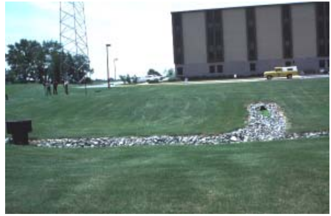
Example of a dry detention facility showing the degree of mowing required and the riprap pilot channel.
