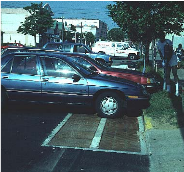
Delaware sand filter.
