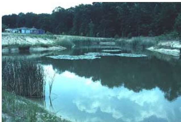
Infiltration basin constructed in the water table. Excellent exfiltration out of the basin sides maintained proper functioning.
