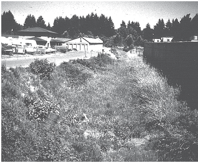
An unmaintained, but well vegetated biofiltration system. Debris needs to be removed from the facility.
