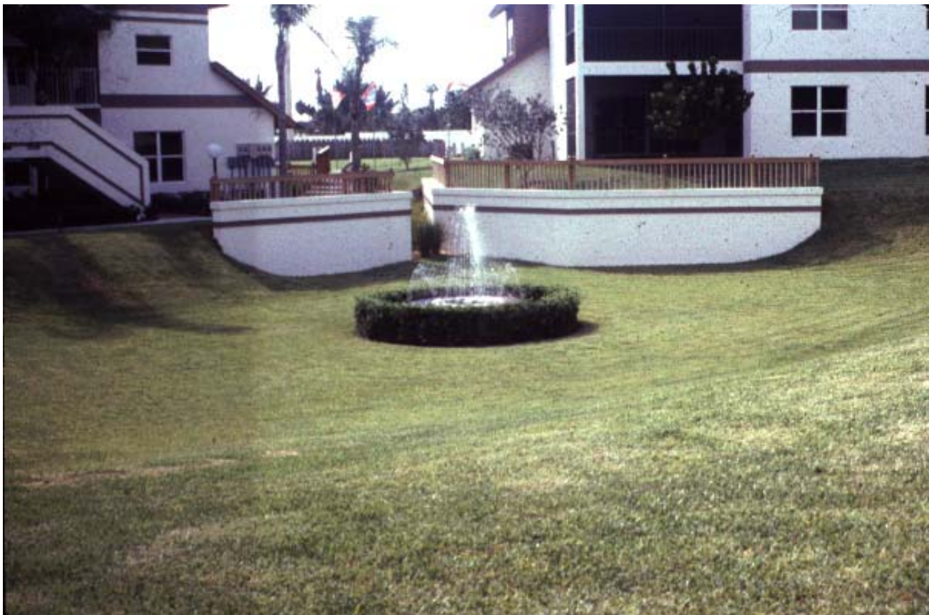
South Florida dry detention system integrated into the site's landscaping.
