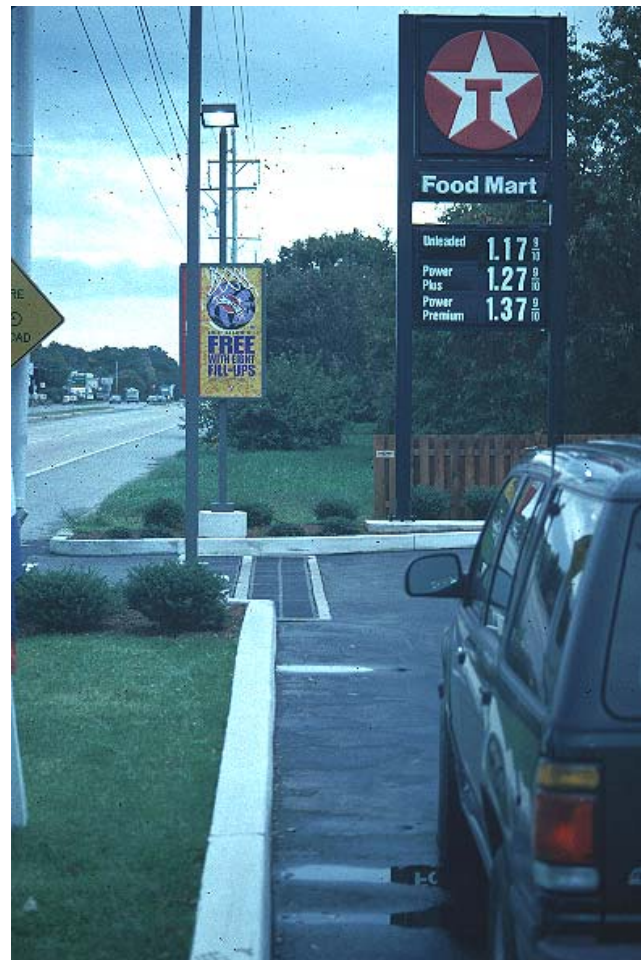
Delaware filtration facility subject to live loads at a gasoline station.
