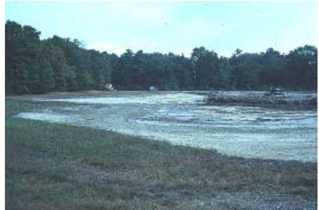
Very shallow grades on a constructed wetland.
